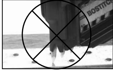
INCORRECT Placement of nail
